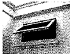
↑ The above casement window, also known as top-hung window, can be commonly found in toilets and above main windows.
