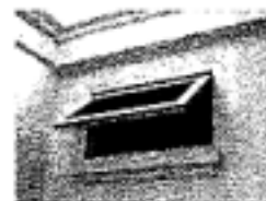
↑ The above casement window, also known as top-hung window, can be commonly found in toilets and above main windows.
